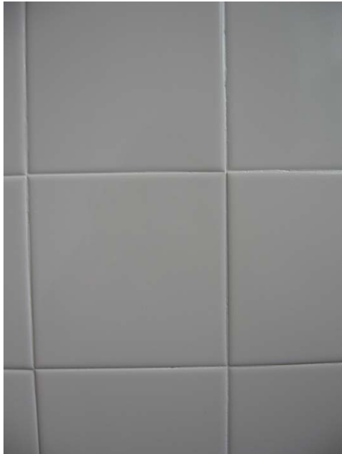
Fig4: Drilled holes and cracks repaired and re-enamelled in high-gloss white
