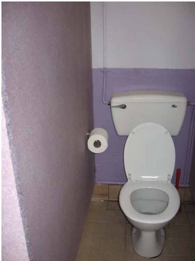
Fig8: Toilets repaired and cubicles resurfaced in fleck granite effect
