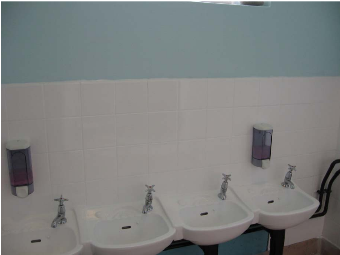
Fig3: Cracked tiles, chipped and tired handbasins re-enamelled in high-gloss white
