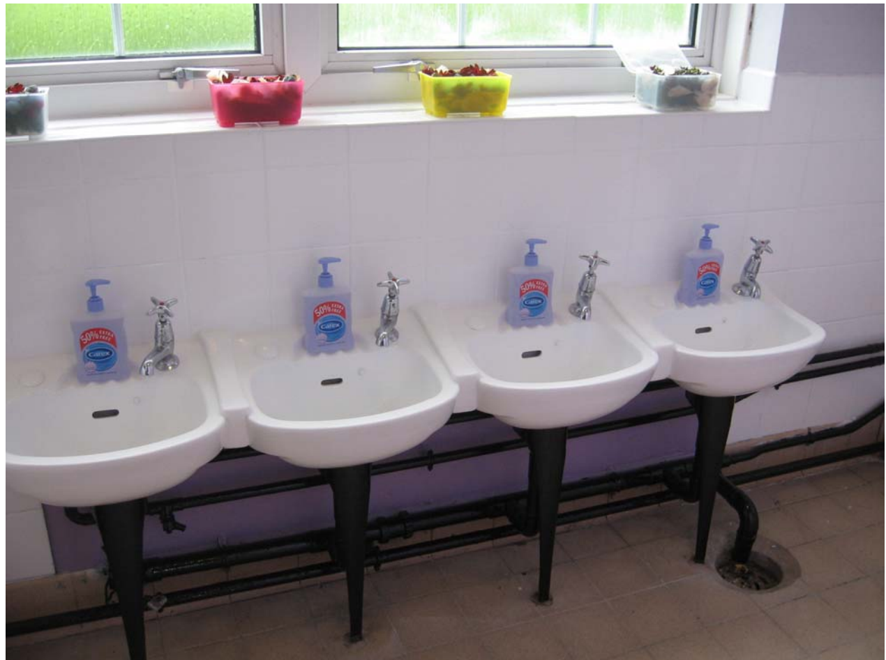
Fig1: Drilled holes/cracks in tiles repaired and handbasins repaired and re-enamelled in high-gloss white
